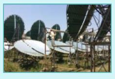
arranged where cooking is done with steam that is generated by solar collectors. Also students got deep knowledge of biogas plant. Air conditioner is also operated by steam that is generated by collectors.
